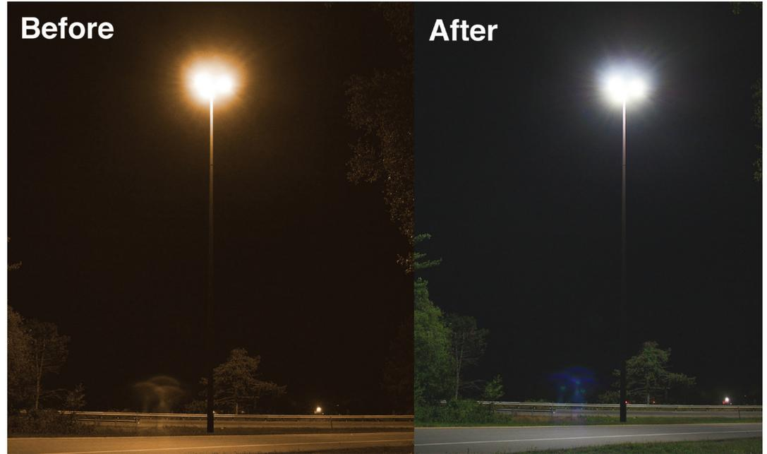
The 3000W HPS (Before) is replaced by the 1000W superior white colour LED (After)
